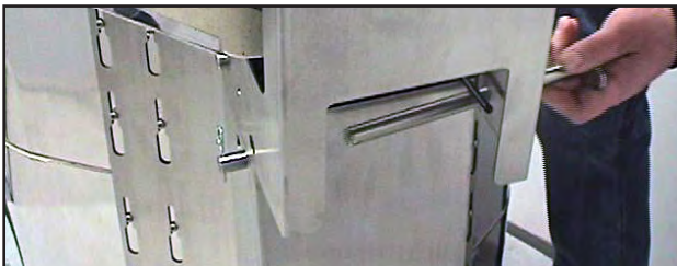
Installing the top-most rod.
